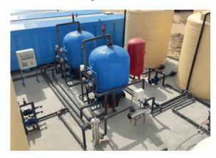
Filtration systems physically separate particles, sand, sediment and organic matter from water. Available in capacities from 0.005 m3/h to 200 m3/h, these systems are used as primary or pre-treatment solutions in plants requiring high quality water. They offer perfect solution to increase the efficiency of filtration, reverse osmosis and deionization systems.
